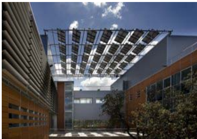
Figure 20. View of the CEDINT/CESVIMA building
